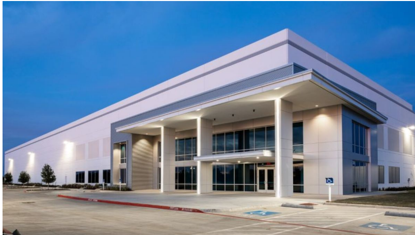
An 800,000-square-foot distribution facility in Fort Worth, Texas. (CoStar)
